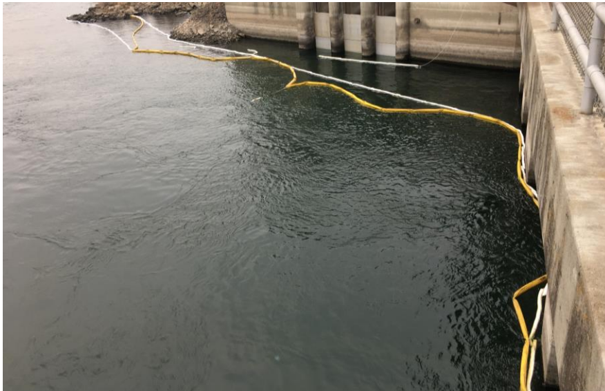
Figure 1. Photo of original absorbent boom deployment on December 7, 2020. Booms were again deployed in this arrangement on January 21, 2021 but no picture was available.
